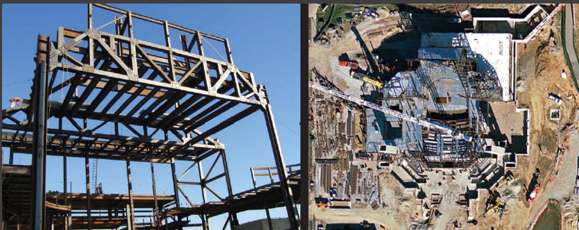
Construction continues to progress at the Carmel Regional Performing Arts Center, Carmel, IN.
