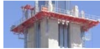
Carillon Tower Cap in Place
